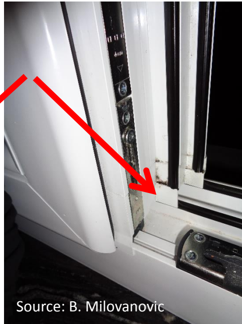
Mold growth due to seal discontinuity
