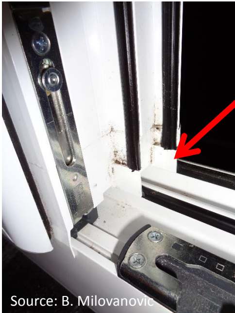
Mold growth due to seal discontinuity
